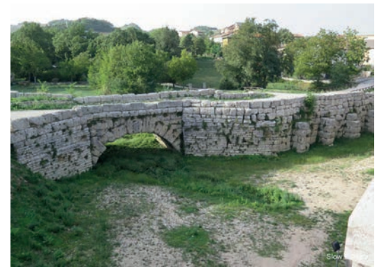
Via Flaminia, the Mallio bridge at Cagli
